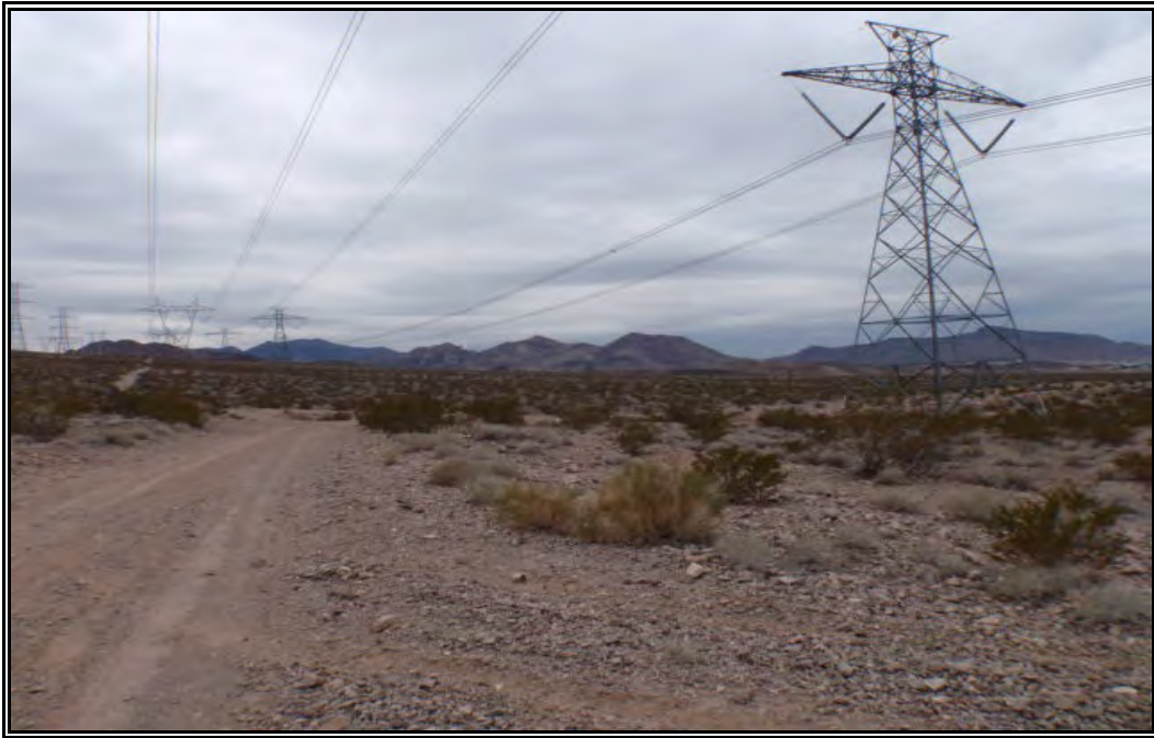
Subject Area Looking West
