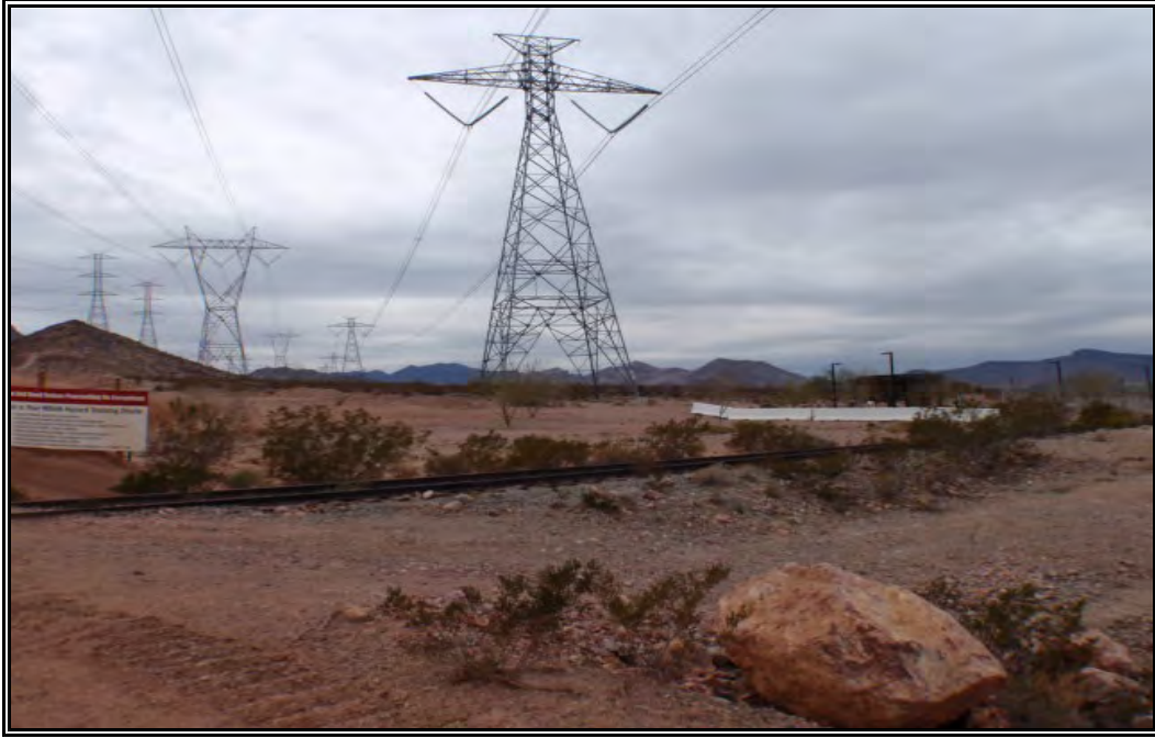
Subject Area Looking West
