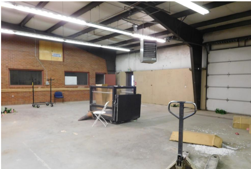
BUILDING 38: TYPICAL INTERIOR VIEW OF STORAGE WAREHOUSE
