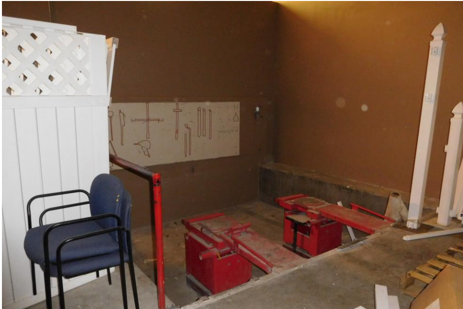
VIEW OF VEHICLE SERVICE PIT LOCATED IN BUILDING 38
