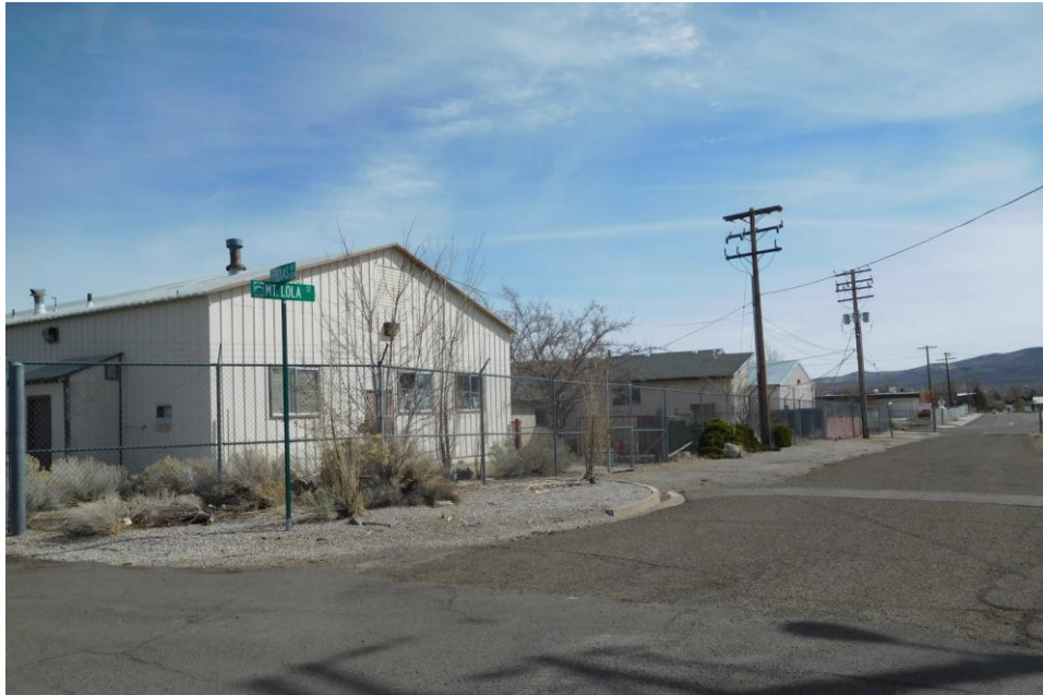
OVERALL VIEW OF SUBJECT PROPERTY FACING SOUTHEASTERLY FROM MT. LOLA STREET AND TEXAS AVENUE
