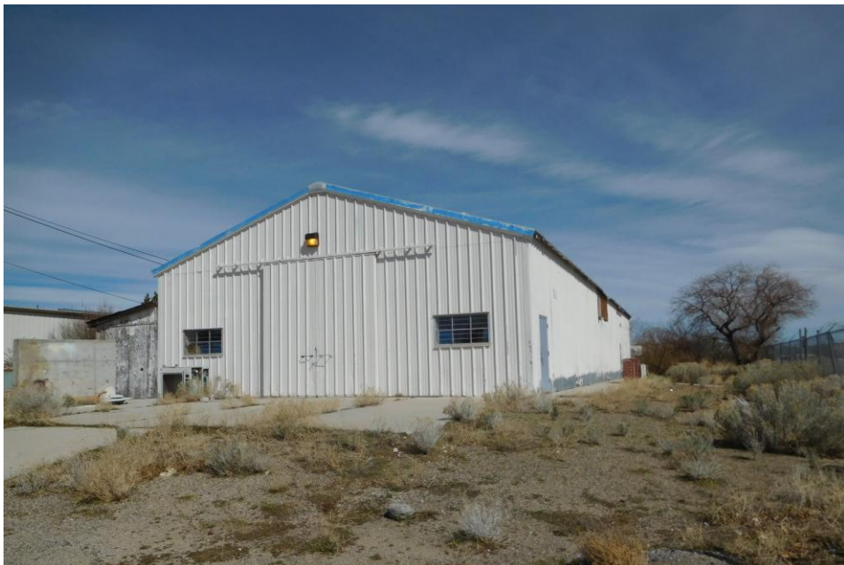
VIEW OF BUILDING 34 (VACANT STORAGE WAREHOUSE)
