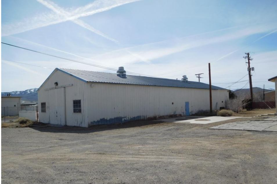
VIEW OF BUILDING 33 (VACANT STORAGE WAREHOUSE)
