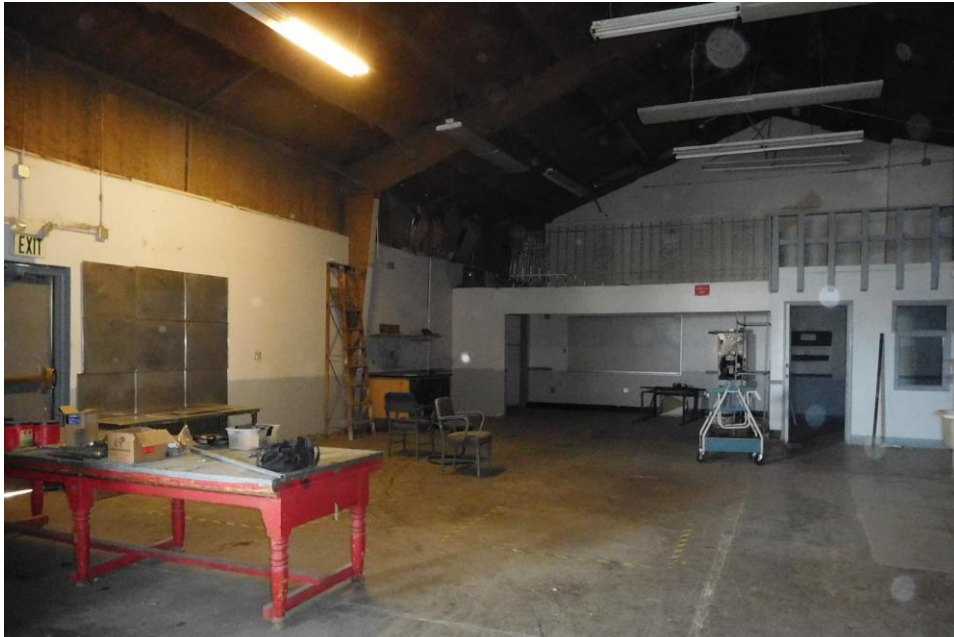
BUILDING 34: INTERIOR VIEW OF SUBJECT WAREHOUSE
