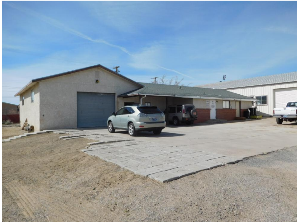
VIEW OF BUILDING 35-A (DRI OFFICE WAREHOUSE)
