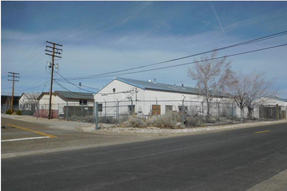
OVERALL VIEW OF SUBJECT PROPERTY FACING NORTHEASTERLY FROM ALPHA AVENUE AND MT. LOLA STREET
