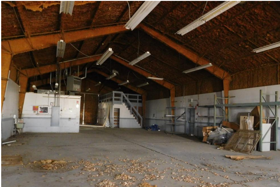
BUILDING 33: INTERIOR VIEW OF SUBJECT WAREHOUSE
