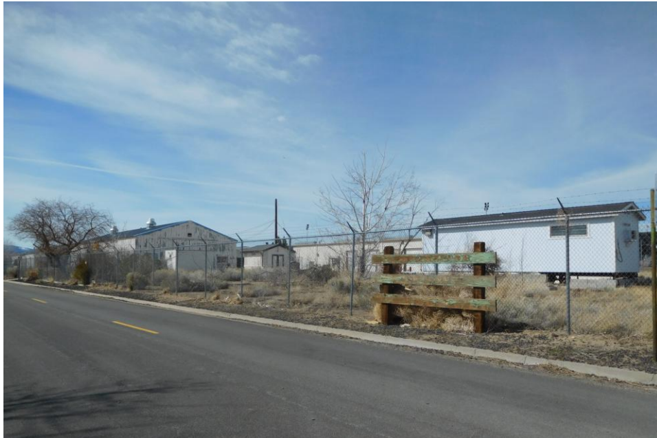
OVERALL VIEW OF SUBJECT PROPERTY FACING NORTHWESTERLY FROM ALPHA AVENUE
