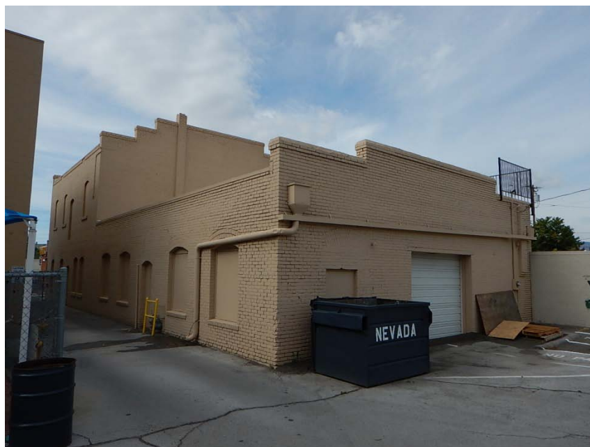
VIEW OF THE STORAGE BUILDING FACING SOUTHWEST
