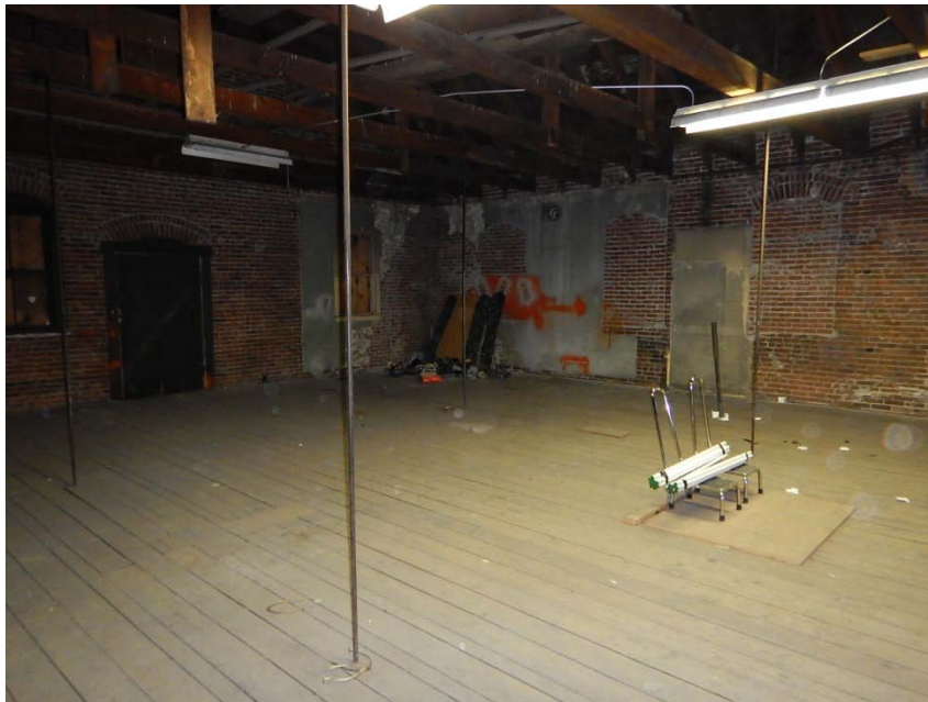
VIEW OF THE SECOND FLOOR INTERIOR OF THE STORAGE BUILDING
