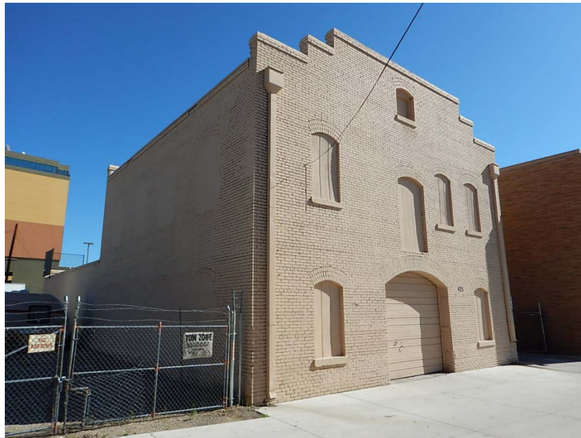
VIEW OF THE STORAGE BUILDING FACING NORTHEAST
