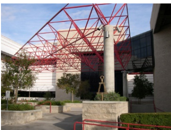
Existing UNLV TBE Building
