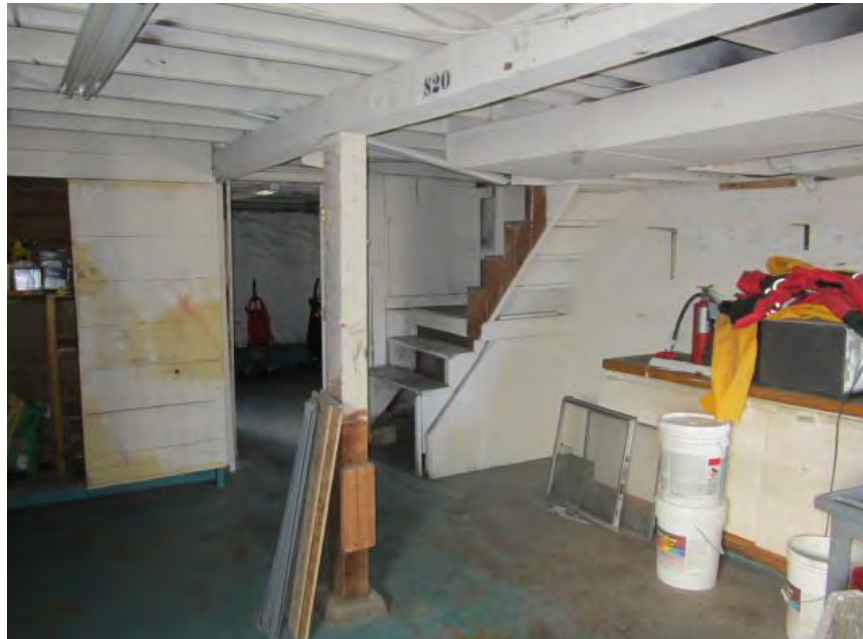
VIEW OF BASEMENT LOCATED IN SUBJECT 4-PLEX
