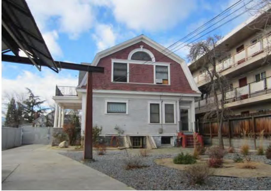
VIEW OF SUBJECT 4-PLEX FACING WESTERLY
