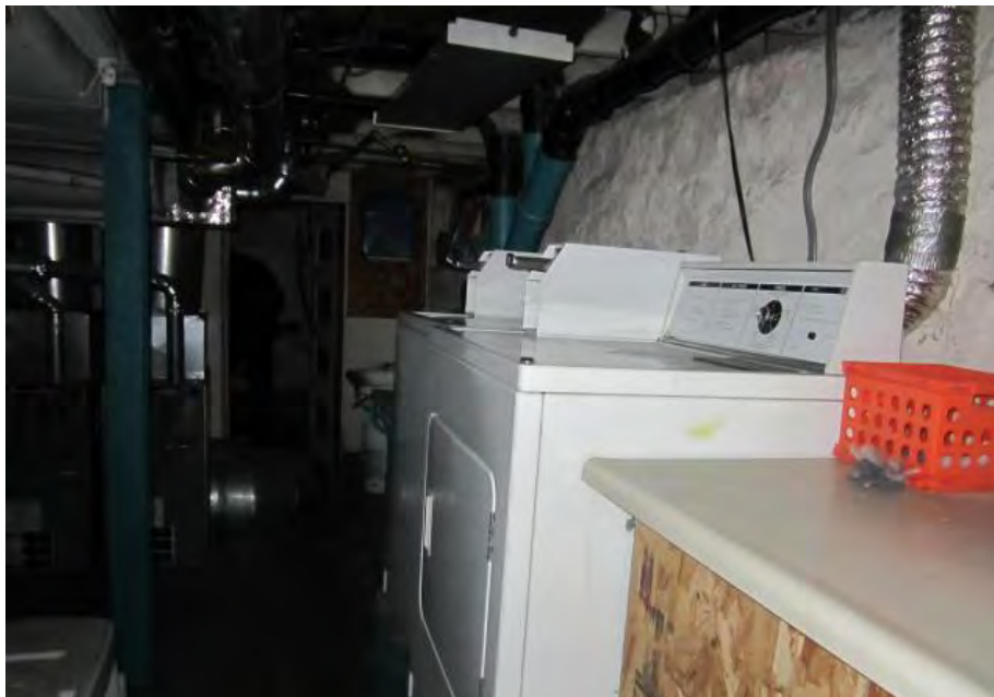
VIEW OF SUBJECT BASEMENT/LAUNDRY AREA
