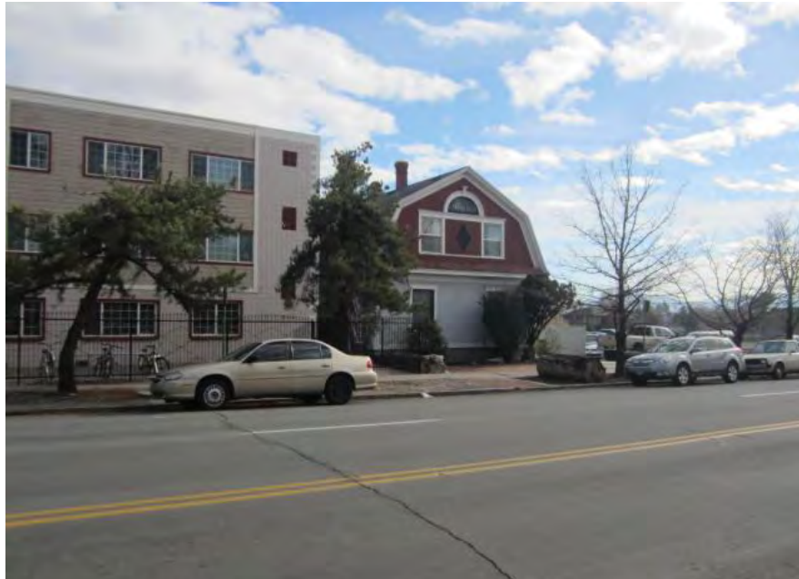
VIEW OF SUBJECT PROPERTY FACING SOUTHEASTERLY FROM NORTH CENTER STREET
