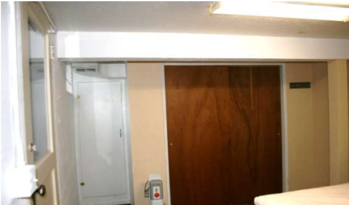
Photograph of southerly basement bedroom area
