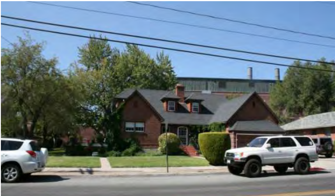
Photograph of front portion of subject property taken from Evans looking westerly
