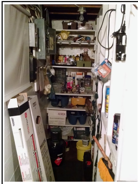
Photograph 6: Additional household chemical storage, including a 5-gallon bucket of concrete sealer.
