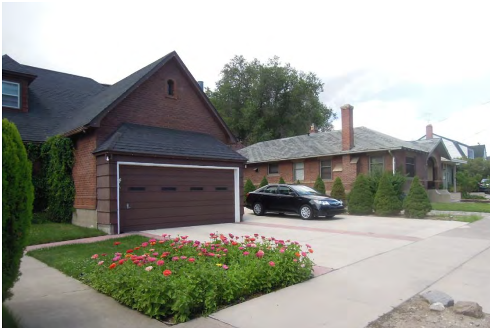
VIEW OF GARAGE AND DRIVEWAY/PARKING PAD
