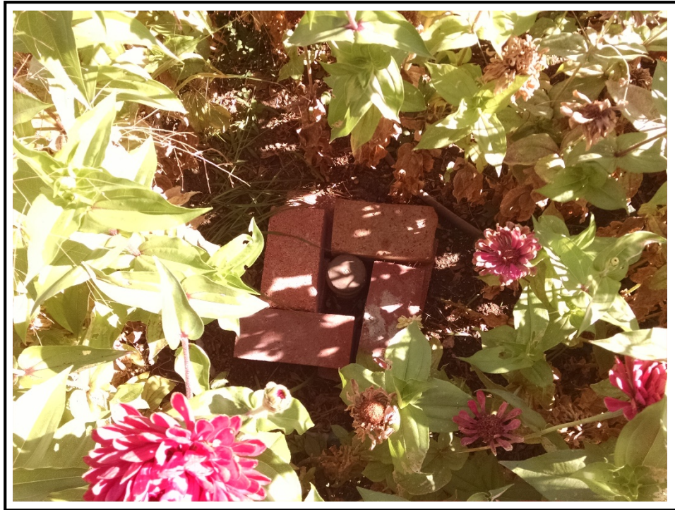
Photograph 3: Fill pipe for heating oil UST, located in the flower bed in the front yard, proximal to the driveway and the sidewalk.
