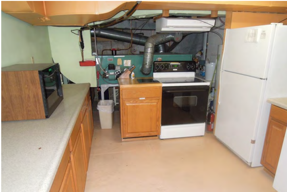
BASEMENT COMMON AREA KITCHEN
