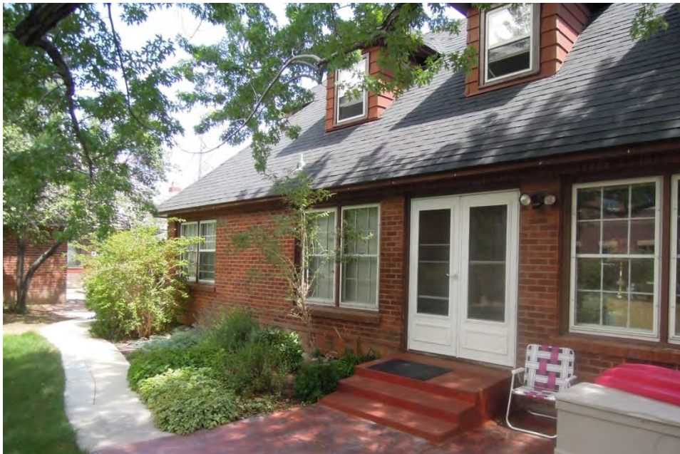
REAR VIEW OF SUBJECT RESIDENCE
