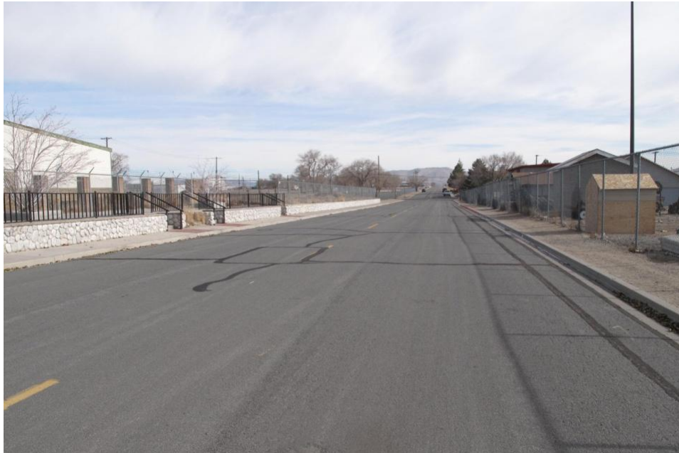
VIEW OF BRAVO AVENUE FACING EASTERLY
