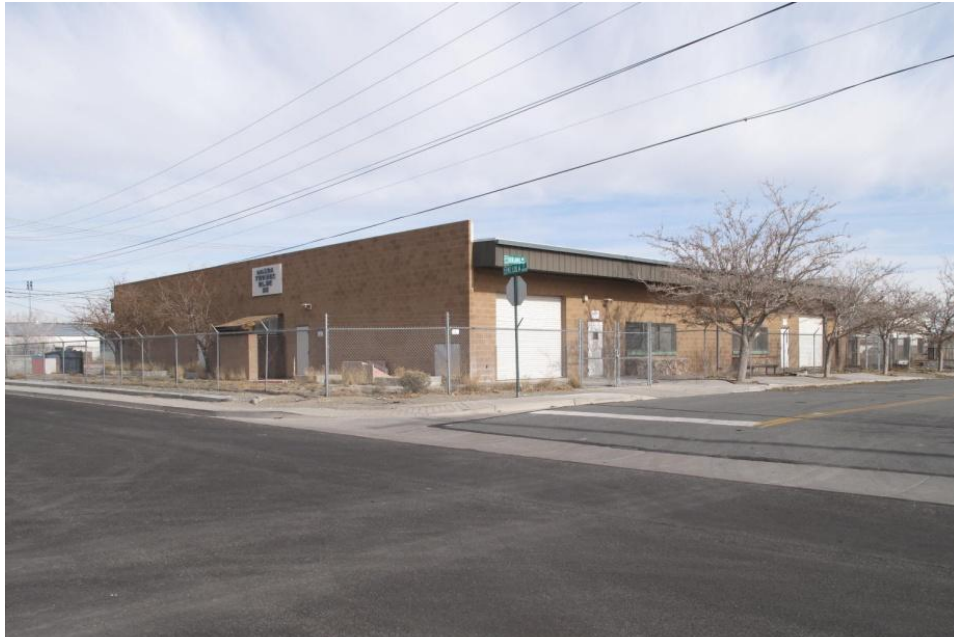
OVERALL VIEW OF SUBJECT INDUSTRIAL FLEX BUILDING FACING NORTHEASTERLY
