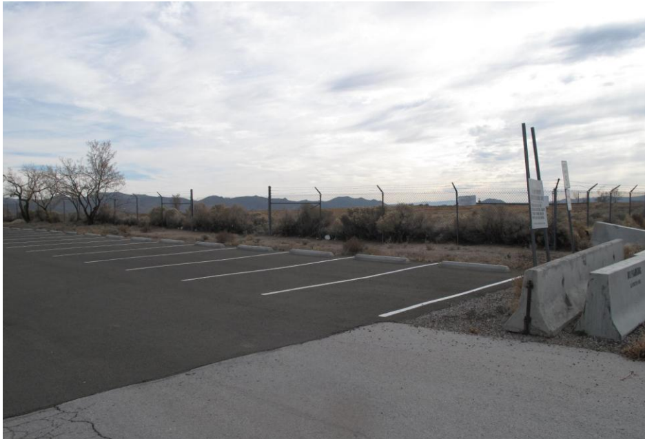
OVERALL VIEW OF SUBJECT PROPERTY FACING IN A SOUTHEASTERLY DIRECTION FROM COCOA AVENUE
