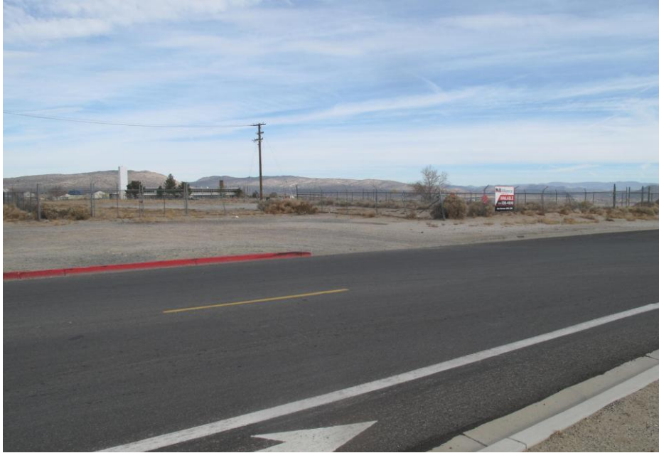
OVERALL VIEW OF SUBJECT PROPERTY FACING NORTHEASTERLY FROM ECHO AVENUE
