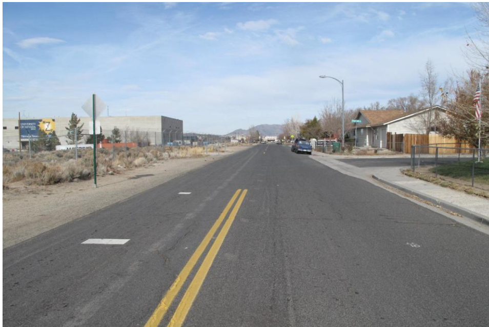
VIEW OF MT. BABCOCK FACING IN A NORTHERLY DIRECTION
