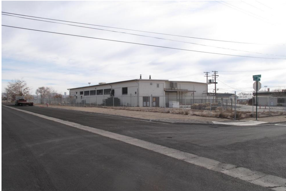
OVERALL VIEW OF SUBJECT PROPERTY FACING IN A SOUTHEASTERLY DIRECTION FROM ALPHA AVENUE AND MT. LOLA
