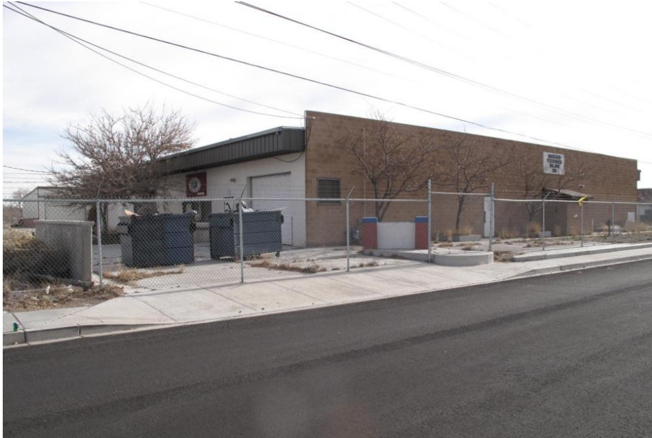
VIEW OF SUBJECT INDUSTRIAL FLEX BUILDING (A.P.N. 086-951-03) FACING IN A SOUTHEASTERLY DIRECTION
