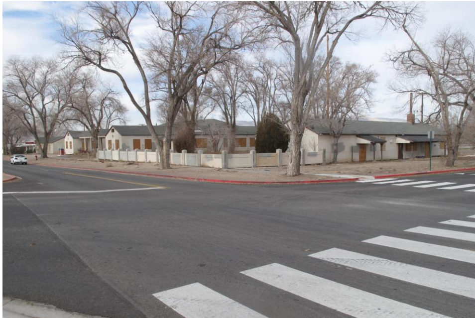
OVERALL VIEW OF SUBJECT PROPERTY FACING IN A NORTHWESTERLY DIRECTION FROM ECHO AVENUE AND MT. VIDA
