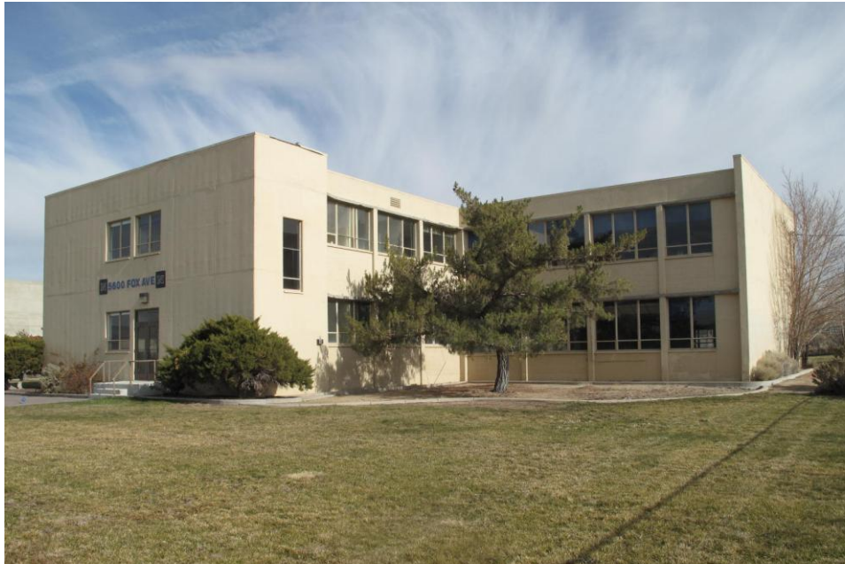
VIEW OF SUBJECT OFFICE BUILDING FACING NORTHEASTERLY
