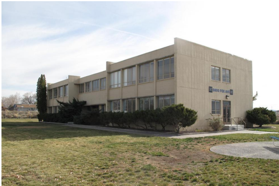
VIEW OF SUBJECT OFFICE BUILDING FACING SOUTHEASTERLY
