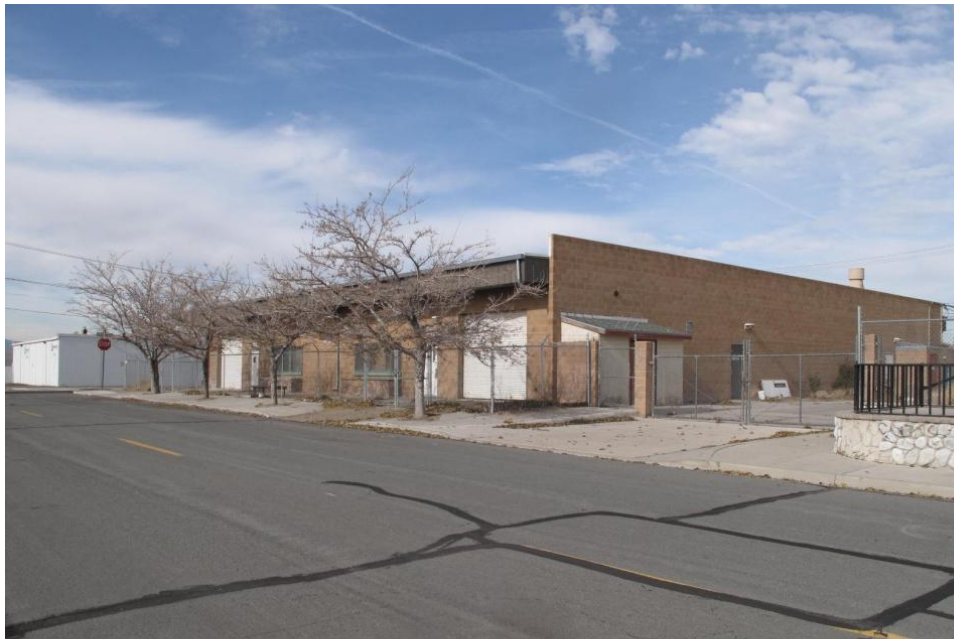
OVERALL VIEW OF SUBJECT INDUSTRIAL FLEX BUILDING FACING NORTHWESTERLY FROM BRAVO AVENUE
