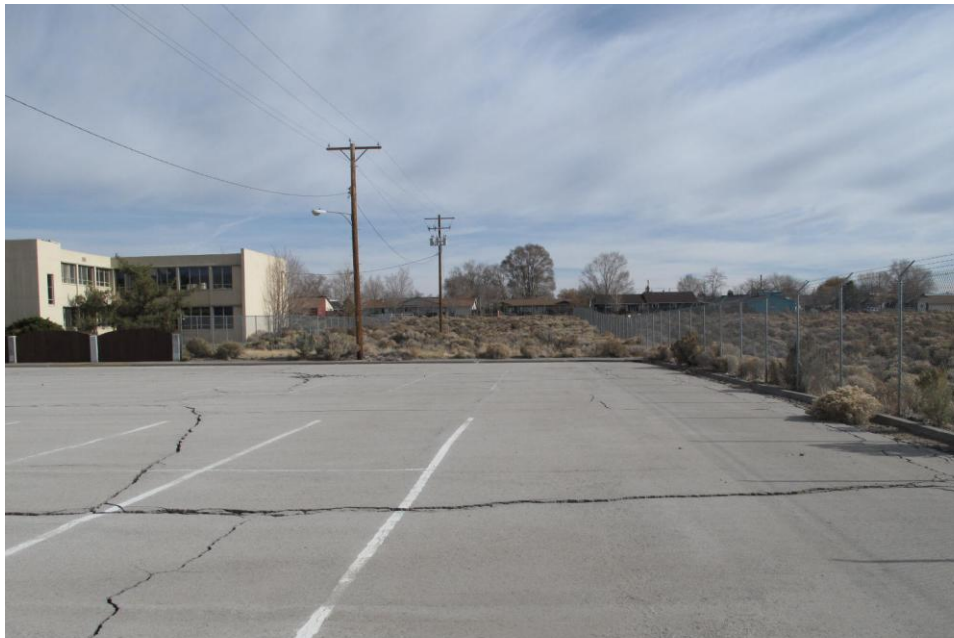
VIEW OF SOUTH SIDE OF SUBJECT PROPERTY (LOCATION OF SURPLUS LAND)
