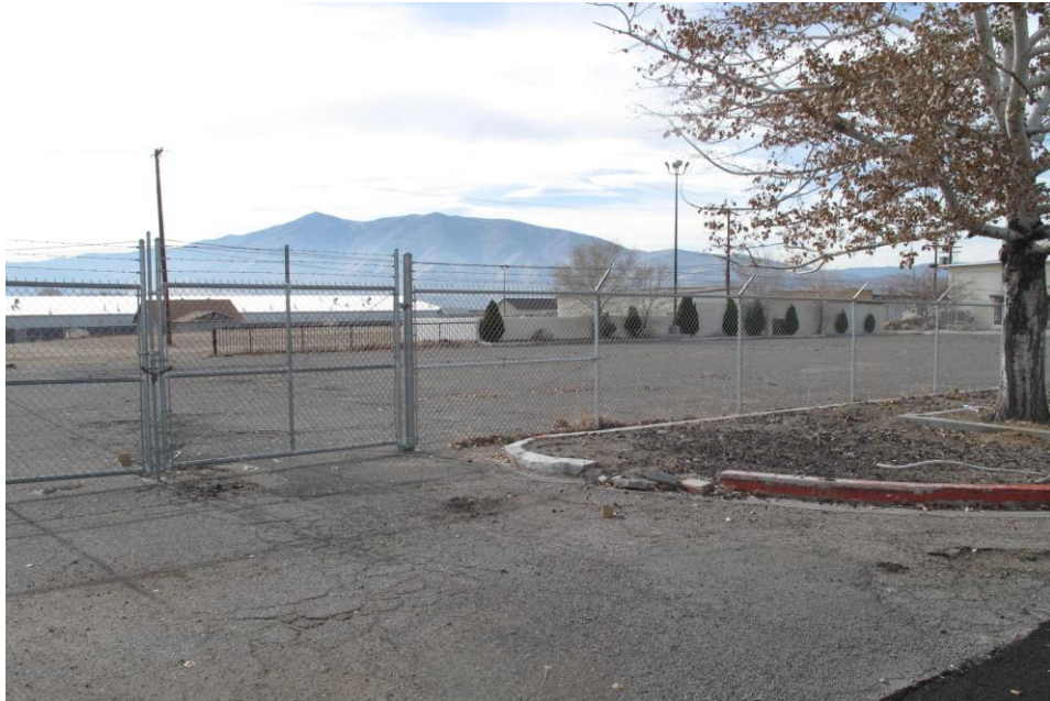
OVERALL VIEW OF SUBJECT PROPERTY FACING IN A SOUTHWESTERLY DIRECTION FROM ALPHA AVENUE
