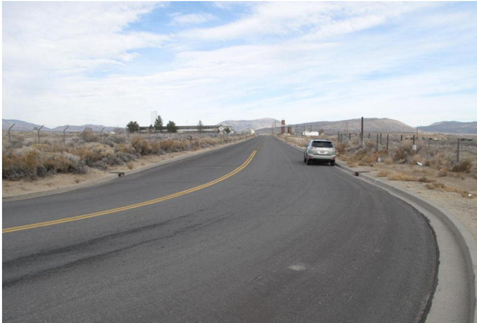
VIEW OF MT. LIMBO FACING NORTHERLY FROM ECHO AVENUE
