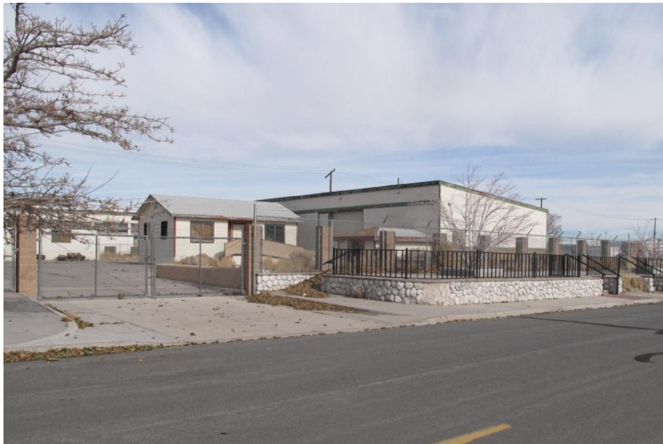
OVERALL VIEW OF STORAGE BUILDING FACING NORTHEASTERLY FROM BRAVO AVENUE
