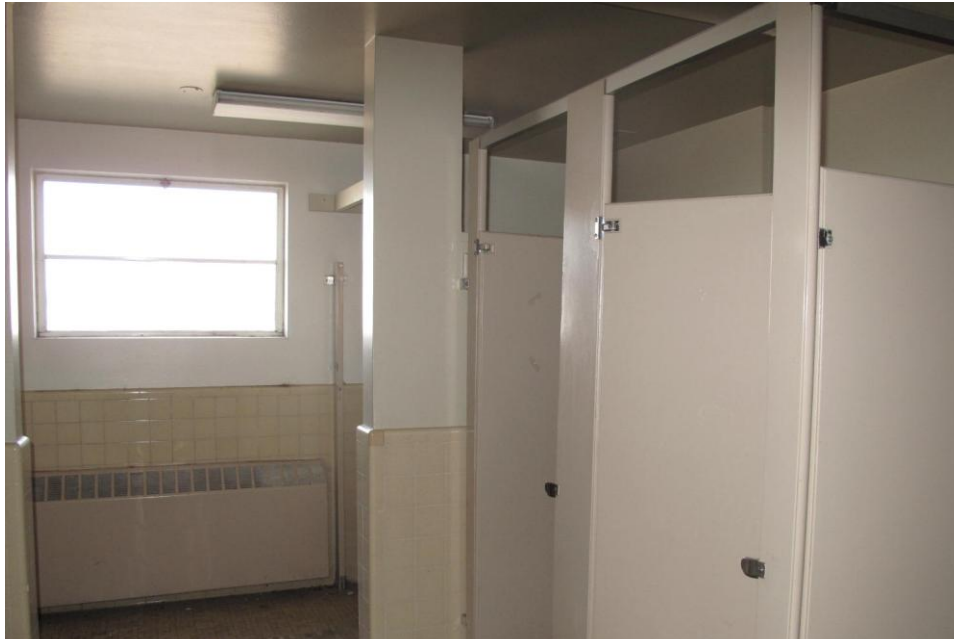
VIEW OF TYPICAL RESTROOM
