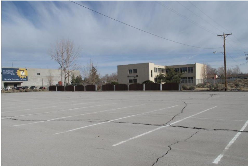
VIEW OF SUBJECT OFFICE BUILDING AND PARKING AREA FACING NORTHEASTERLY
