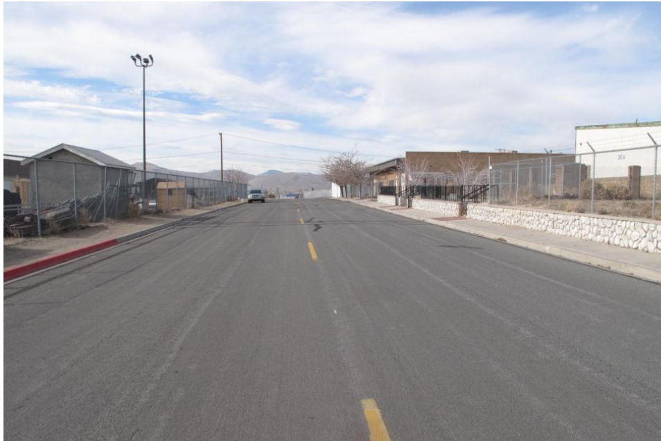
VIEW OF BRAVO AVENUE FACING WESTERLY
