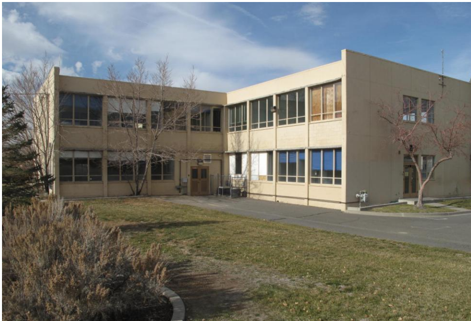
VIEW OF SUBJECT OFFICE BUILDING FACING NORTHWESTERLY
