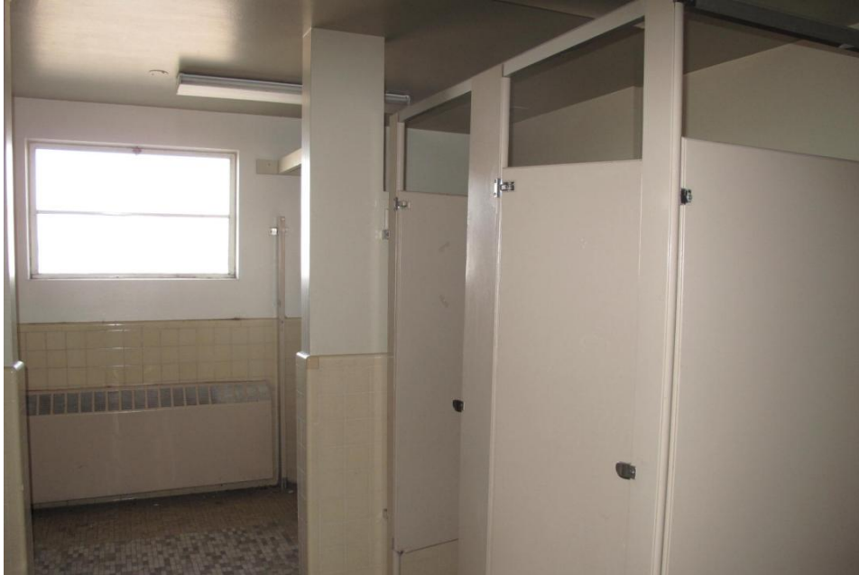
VIEW OF TYPICAL RESTROOM
