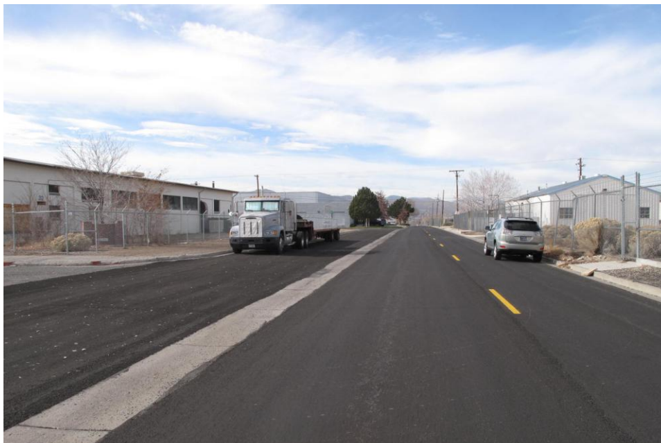
VIEW OF ALPHA AVENUE FACING IN A WESTERLY DIRECTION
