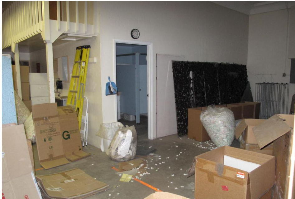
VIEW OF TYPICAL RESTROOM IN SUBJECT INDUSTRIAL FLEX BUILDING
