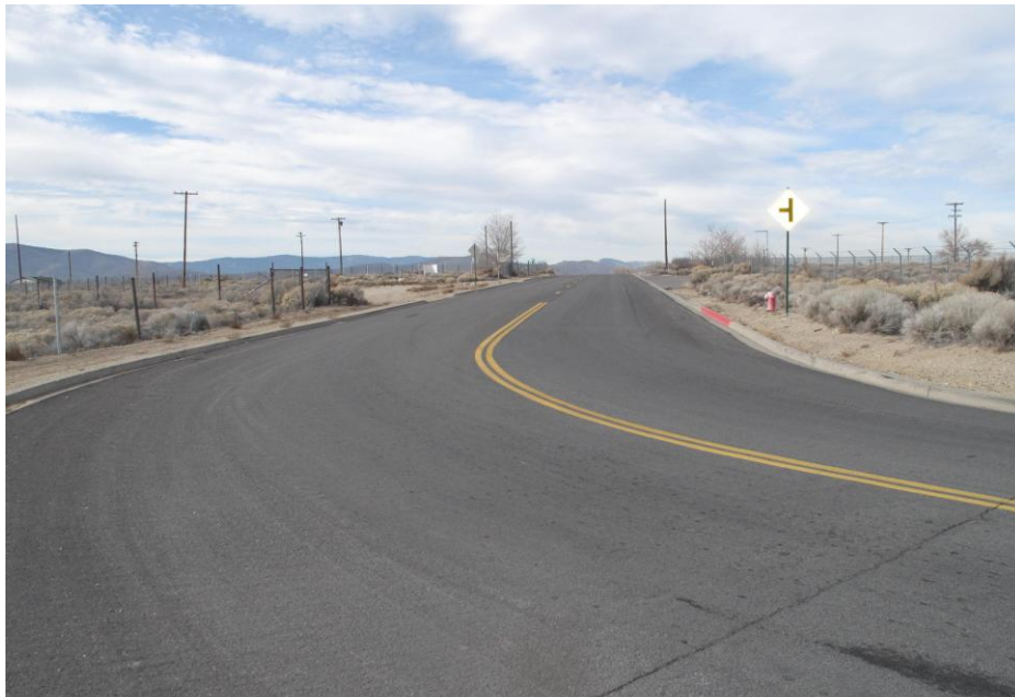
VIEW OF ECHO AVENUE FACING IN A WESTERLY DIRECTION FROM MT. LIMBO
