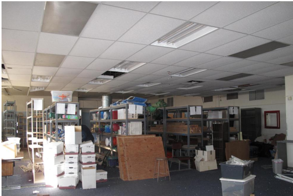
VIEW OF TYPICAL STORAGE SPACE
