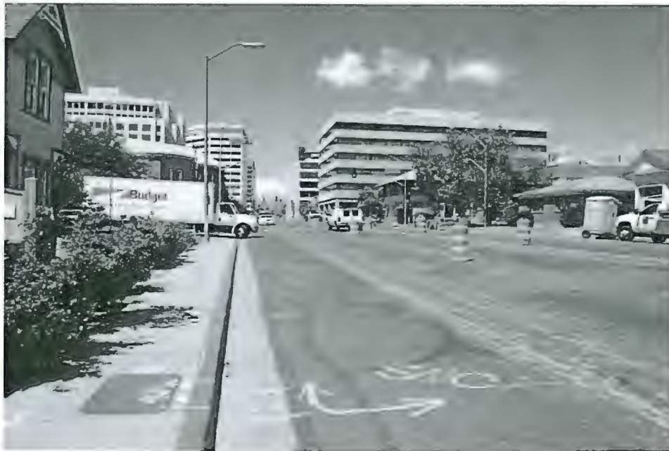
VIEW OF EAST LIBERTY STREET FACING WEST IN THE VICINITY OF THE SUBJECT PROPERTY
