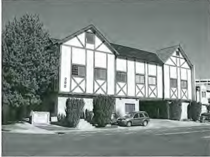
Comstock Building 295 Holcomb Avenue
