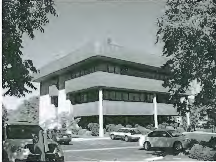
Holcomb Professional Center 333 Holcomb Avenue
