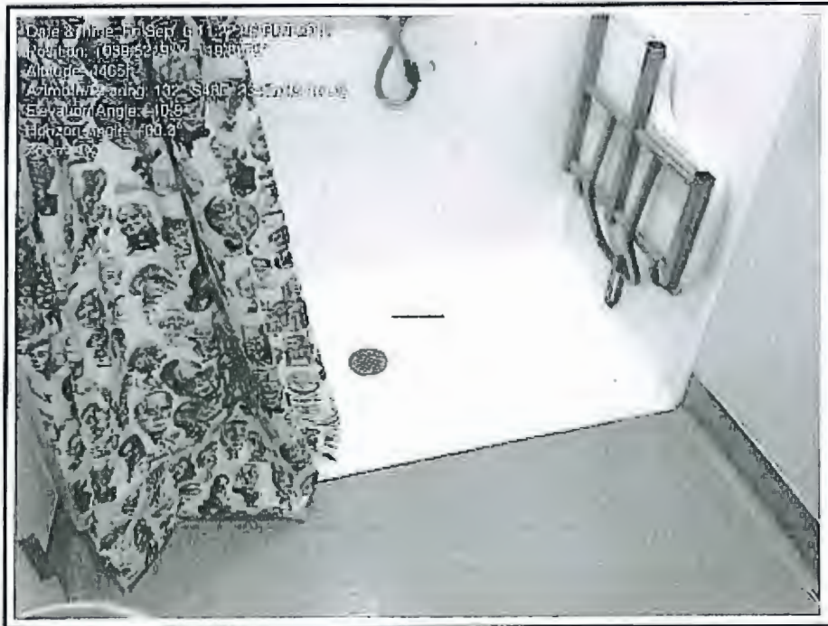
Photograph 24: View of observed shower room within the basement of the building
